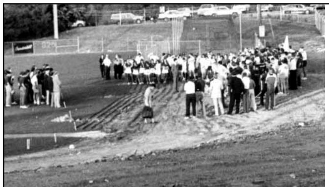
Team and school officials gathered at Dudy Noble Field on May 4, 1986 to break ground on the new grandstand. Demolition crews needed less than a week to remove the old grandstand and ready the site for construction.
